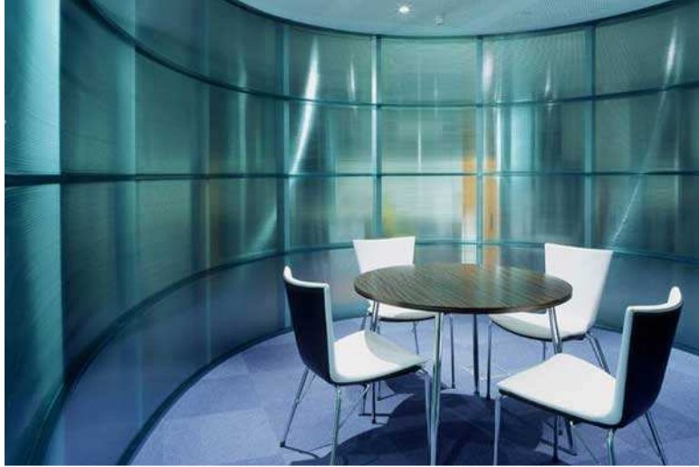
Figure 6. Office with walls made from polycarbonate.
